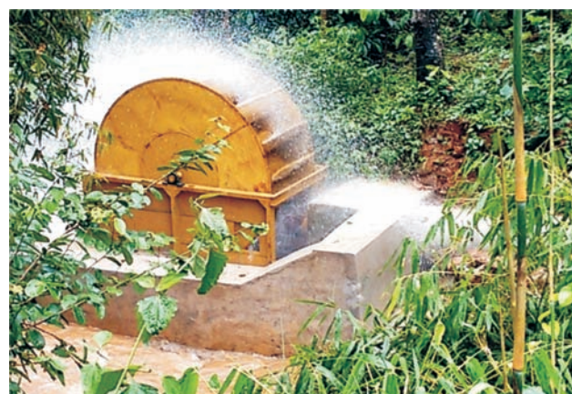
Modified Hydro Electric Turbine, developed by the author, in action
